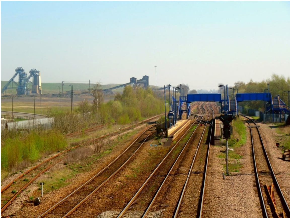
Hatfield and Stainforth Railway Station (Right) with Hatfield Main Colliery Head Gears and Conveyor system (Left), Stainforth
